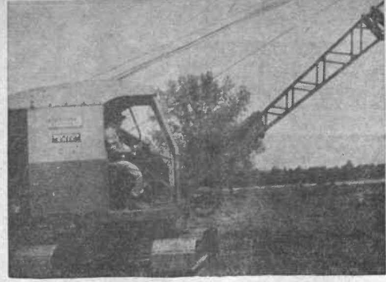
DRAGLINE REPLACES HAND SHOVEL—Digging ditches on farm land in Tishomingo County is done quickly and efficiently with the dragline. The above photo shows the operator digging a ditch which has been surveyed by local Soil Conservation Service personnel on James S. Kimbrough's farm northwest of Burnsville.
